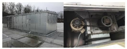
Figure II - Package DX Cooling
